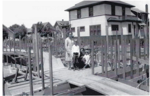
Construction site with parsonage in background
