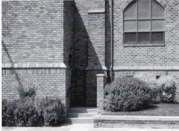
Side Entrance Before Elevator Addition
