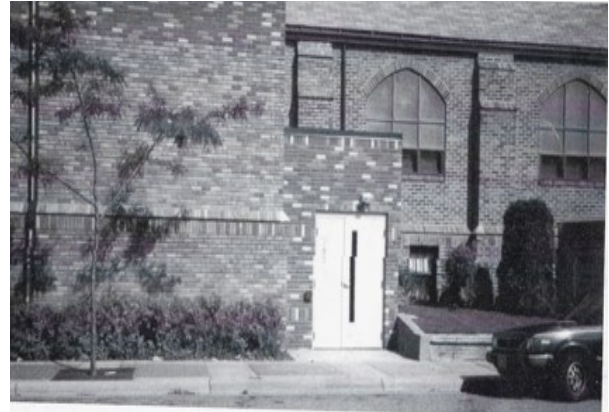
Side Entrance After Elevator Addition
