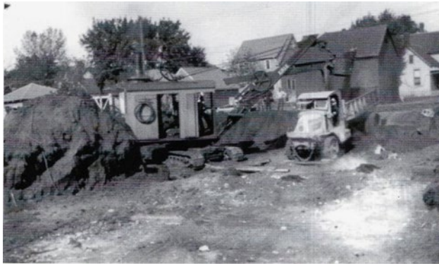
Excavation of new church site 1928
